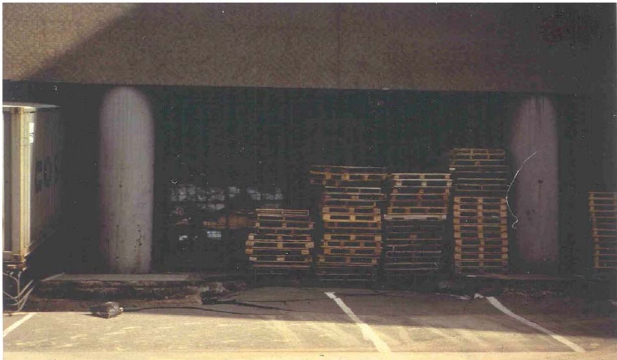
Differential Settlement Between Building on Piles and Natural Ground Caused by Liquefaction and Compaction of Artificial Fill during the 1995 Kobe, Japan Earthquake
