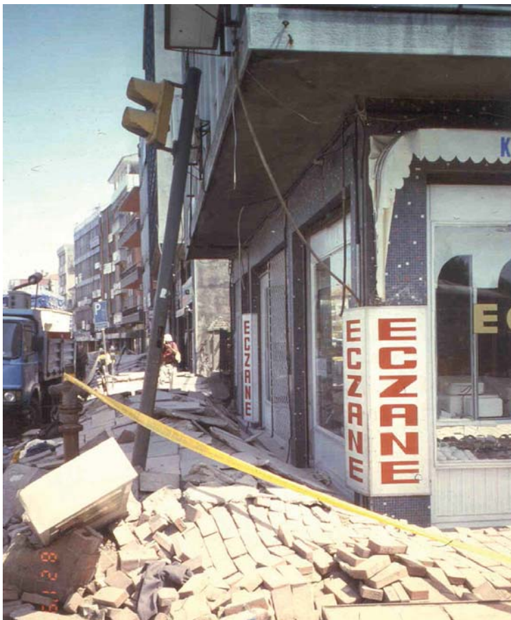
Building Settlement in Adapazari, Turkey Caused by Liquefaction-Induced Loss of Bearing Strength during 1999 Koaceli, Turkey Earthquake
