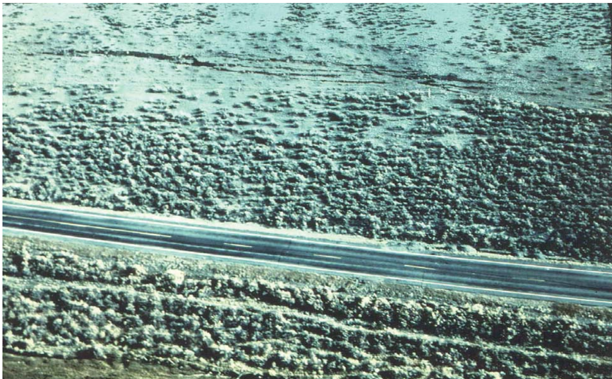
Whiskey Springs Lateral Spread Generated by the 1983 Borah Peak Earthquake Displaced Highway 93 1 m toward Camera
