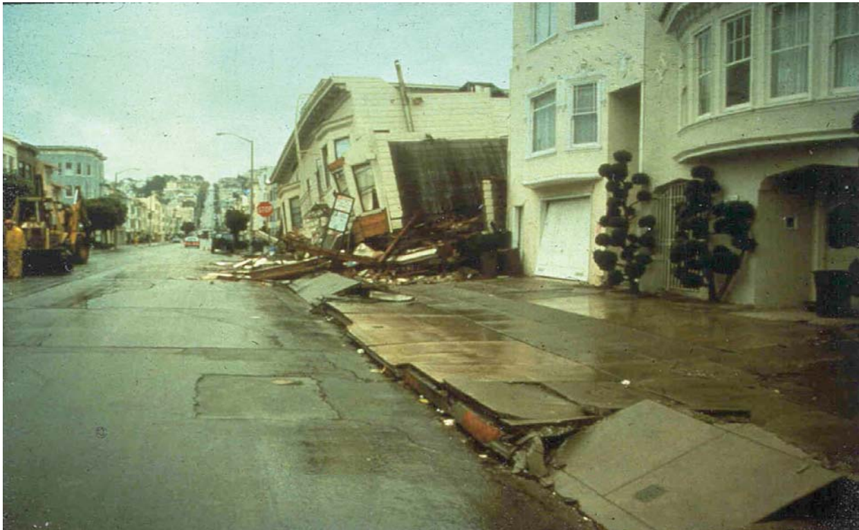
Walk and Curb Damage Caused by Ground Oscillation (1989 Loma Prieta, Calif. Earthquake)
