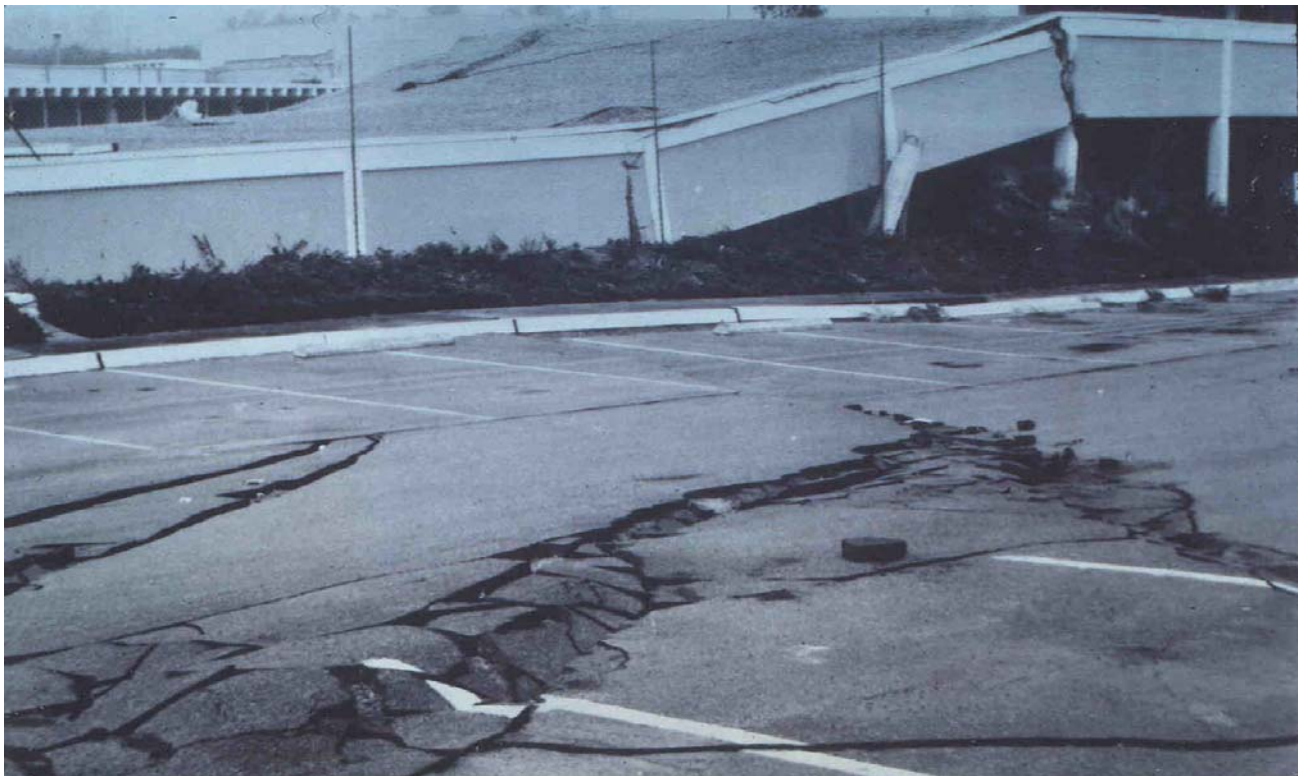
San Fernando Valley Juvenile Hall Damaged by Lateral Spread During 1971 San Fernando, Calif. Earthquake
