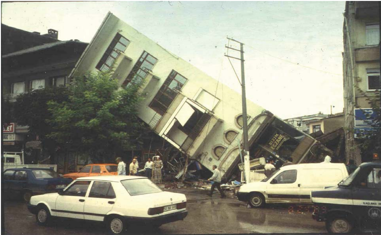
Tipped Building in Adapazari, Turkey Caused by Liquefaction-Induced Loss of Bearing Strength during 1999 Koaceli, Turkey Earthquake
