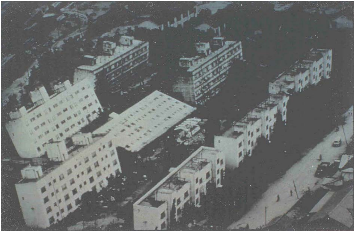
Tipped Buildings Caused by Liquefaction-Induced Loss of Bearing Strength, 1964 Niigata, Japan Earthquake
