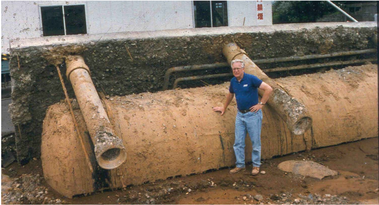
Oil Tank that Buoyantly Floated to Ground Surface through Liquefied Soil during 1983 Hokkaido-Nansei-Oki, Japan Earthquake
