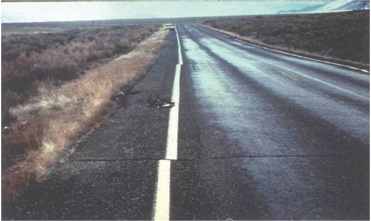
Segment of Highway 93 Displaced 1 m to Left by Whiskey Springs Lateral Spread; 1983 Borah Peak, Idaho Earthquake
