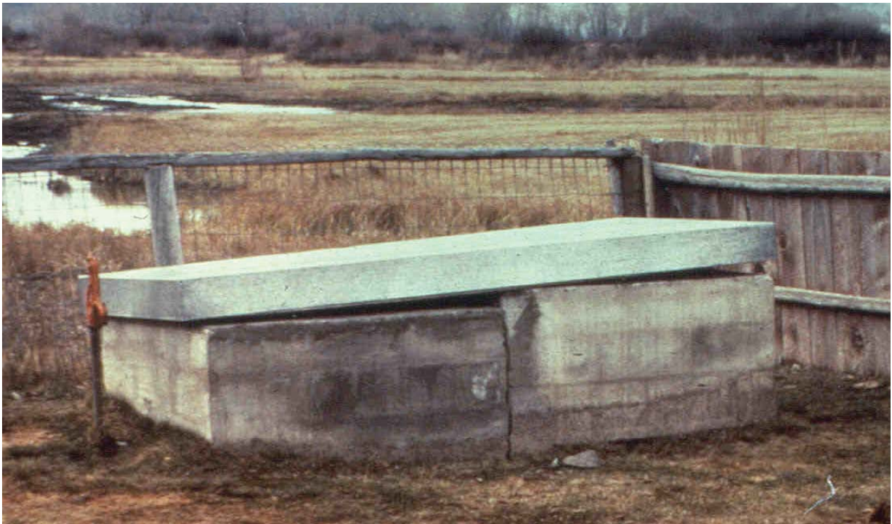
Water Tank on Right Buoyantly Rose Due Liquefaction of Subsurface Soils at Pence Ranch; 1983 Borah Peak Earthquake
