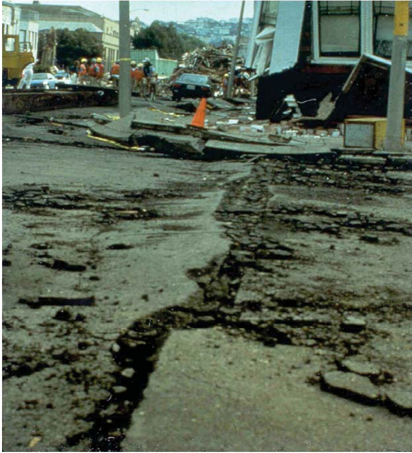
Pavement and Curb Damage Caused by Ground Oscillation during 1989 Loma Prieta, Calif. Earthquake
