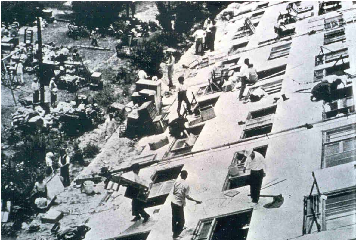
Tipped Buildings Caused by Liquefaction-Induced Loss of Bearing Strength, 1964 Niigata, Japan Earthquake Courtesy of Professor T. L. Youd
