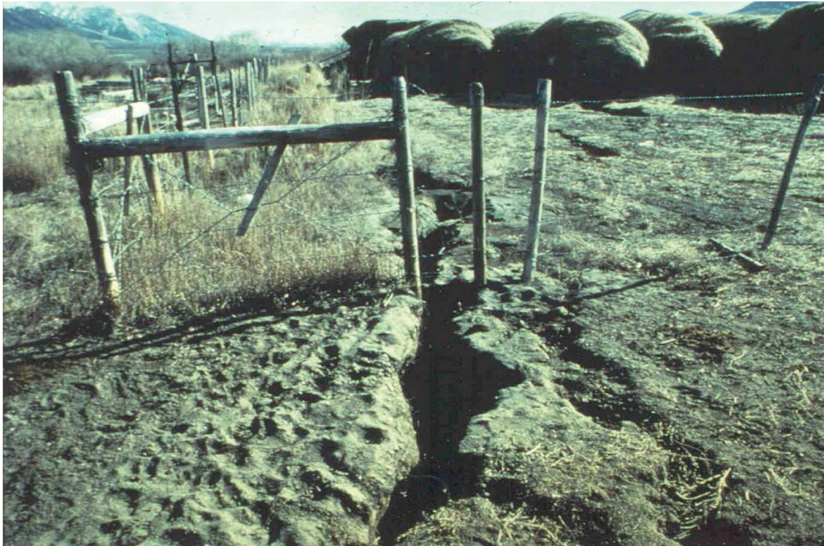
Fence on Pence Ranch Pulled Apart by 0.45 m Due to Lateral Spread During 1983 Borah Peak, Idaho Earthquake
