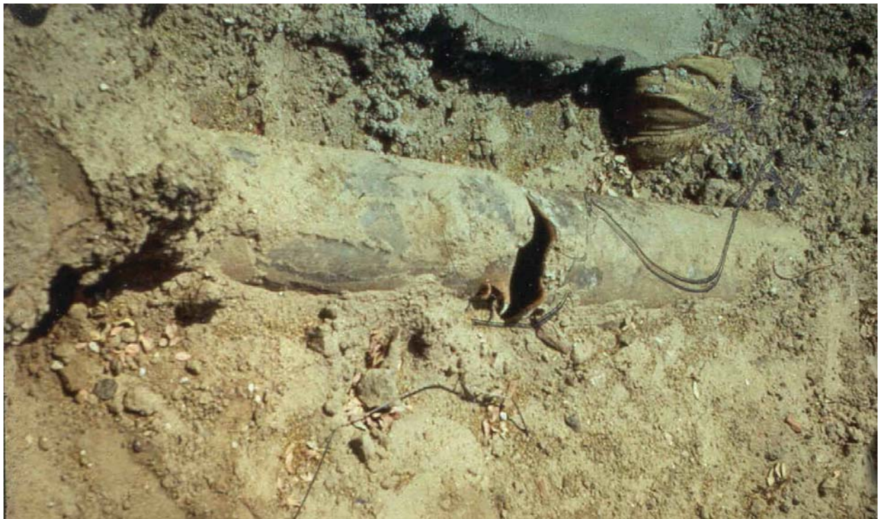
Water Pipeline Break Caused by Displ. of San Fernando Valley Juvenile Hall Lateral Spread
