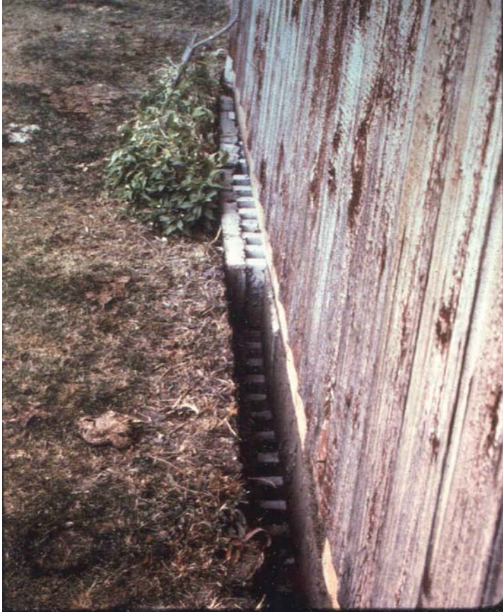
View of Back of House on Pence Ranch Showing Wall Pulled Away from Foundation because of Lateral Spread; 1983 Borah Peak, Idaho Earthquake
