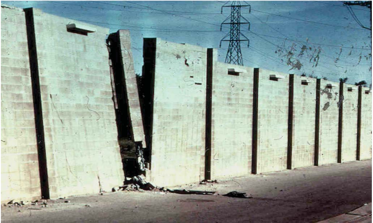
Wall around San Fernando Valley Juvenile Hall Was Pulled Apart by Lateral Spread during 1971 Earthquake
