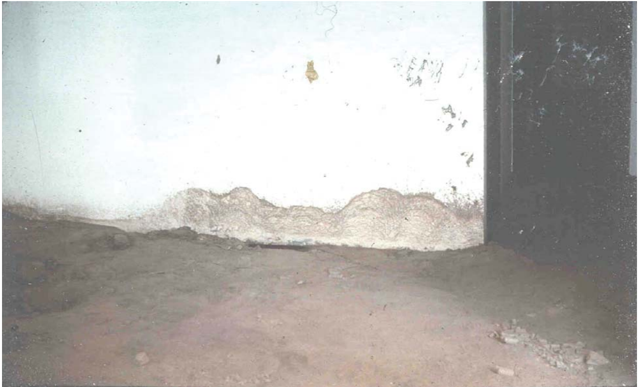
Sand Boil Erupted within House in Caucete during the 1977 San Juan, Argentina Earthquake
