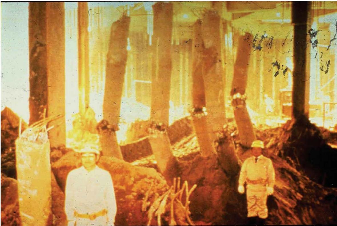
Fractured Piles Beneath Building Caused by Lateral Spread (1964 Niigata, Japan Earthquake)
