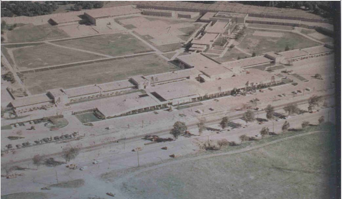
San Fernando Valley Juvenile Hall Damaged by Lateral Spread During 1971 San Fernando, Calif. Earthquake
