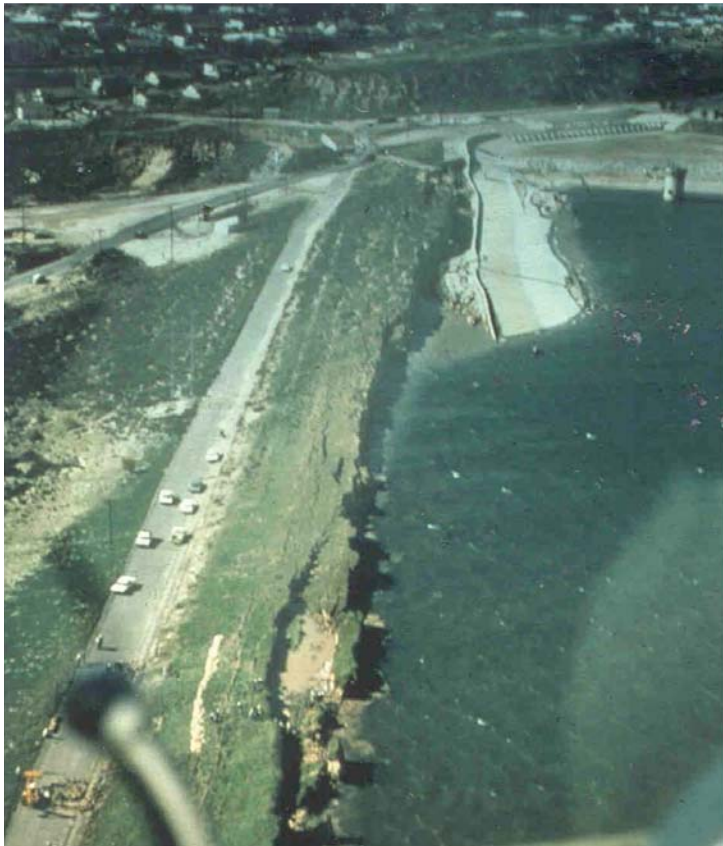
Crest and Upstream Embankment of Lower San Fernando Dam Slipped Upstream and into Reservoir Due to Liquefaction-Induced Flow Failure During 1971 San Fernando, California Earthquake
