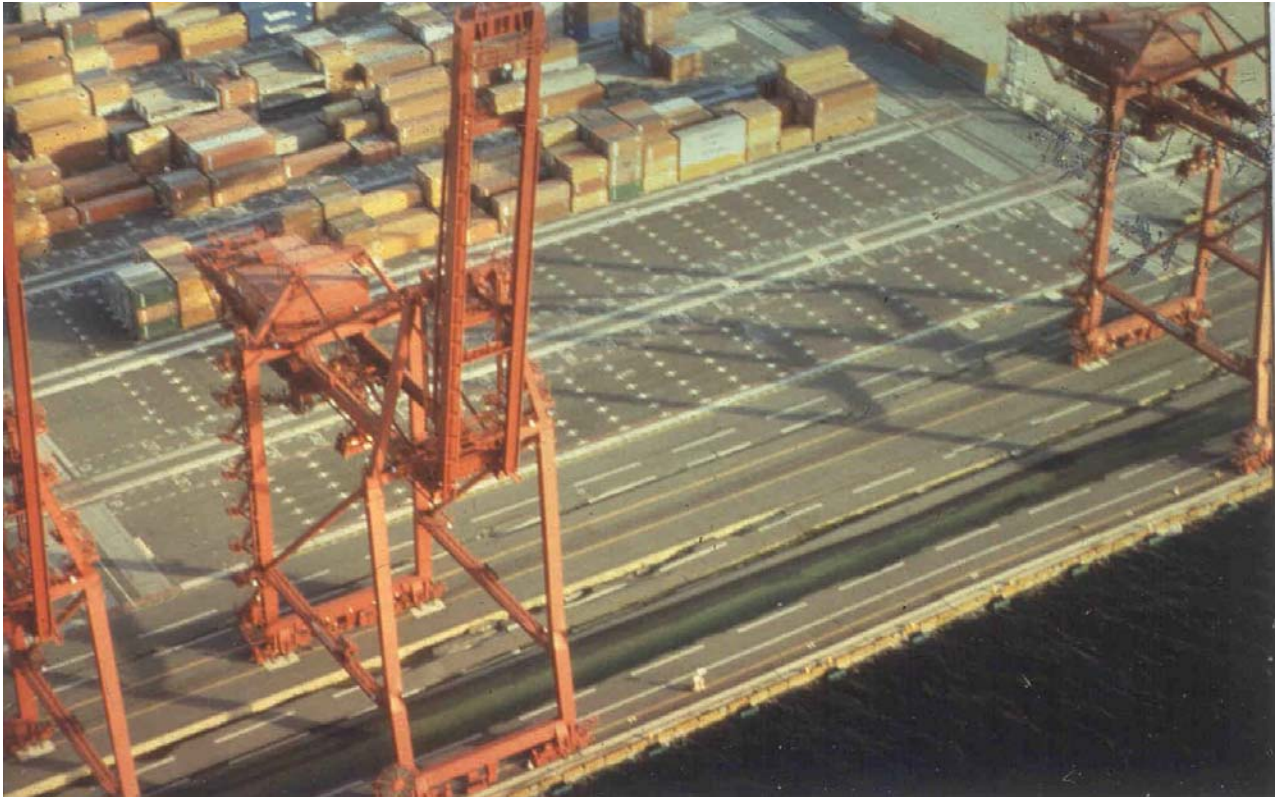
Crane Legs Pulled Apart and Buckled by Lateral Spread Displacement
